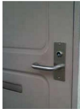
Replacement of door knob with lever handle
