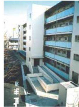
Installation of ramp
