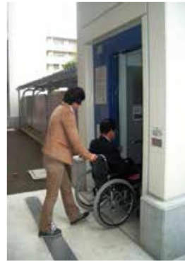
Installation of elevator
