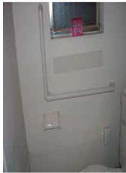
Installation of handrail
