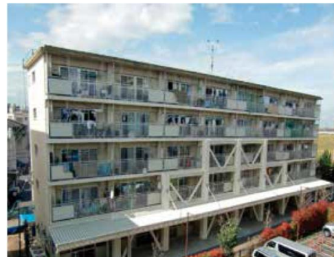
Bracing installed on the balcony side
