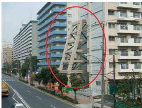
Installation of buttress on the gable wall
